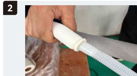
2 Connect the drain pipe to the indoor drain outlet.
