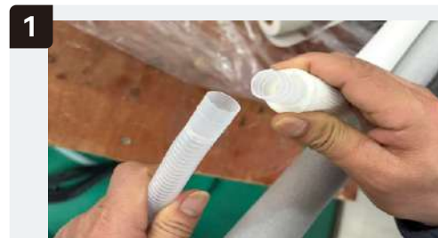
1 Locate the larger end of the drain hose and prepare it for connection.
