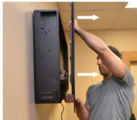
b. pull glass panel away from wall
